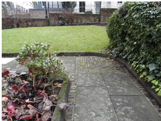
Some of the retained brickwork and materials
